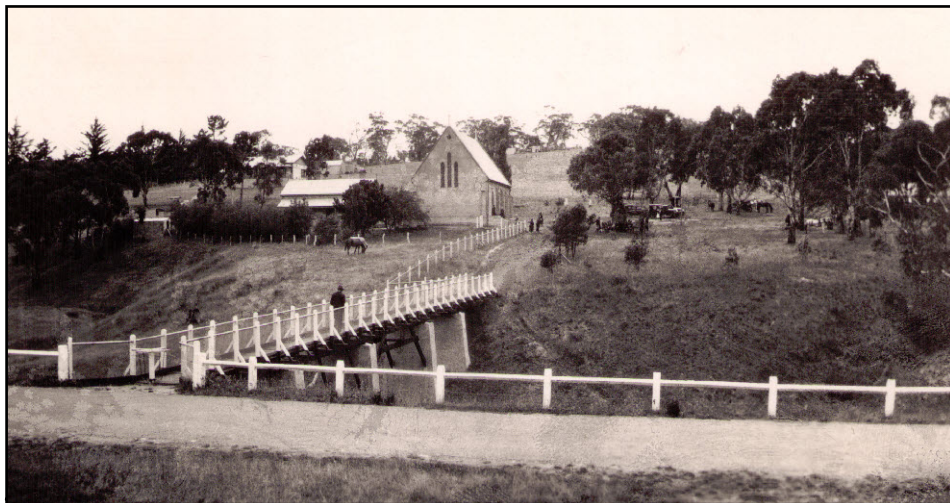
St. James The Less Catholic Church and footbridge c1936.
